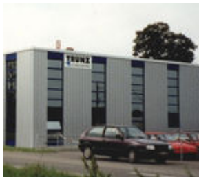
1995 Foundation of air duct system, Langenthal
