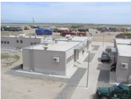
The Trunz Water System provides cleaning water for the truck driver camp.
