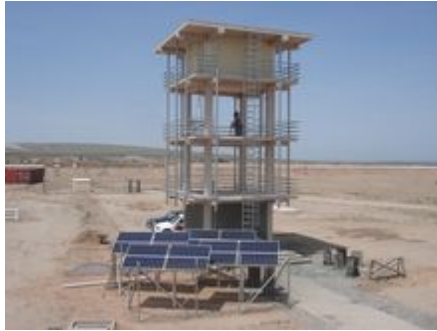
Our solution pumps water from the river about 1km in underground pipes to the central water station.
